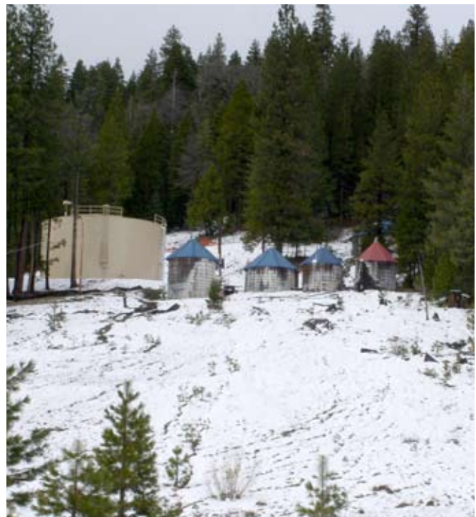
Mineral, California was able to upgrade its water storage system through funding from bank, nonprofit, and government sources.
